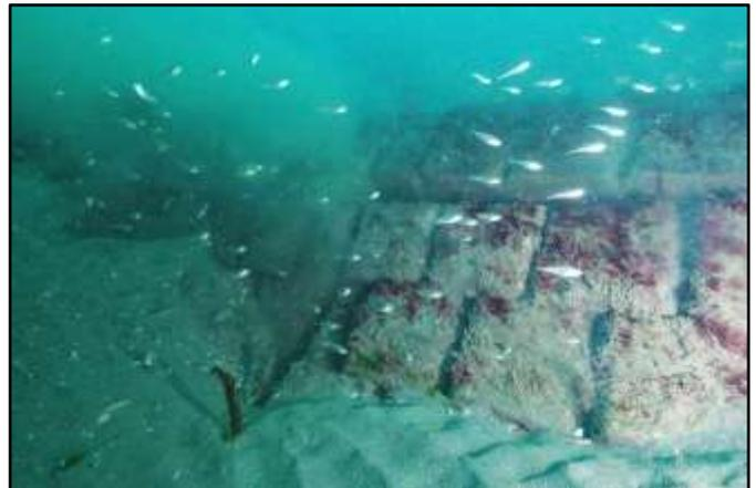
**Plate 13.2.** Leaking sewer pipe at Cheyne Cove, Ilfracombe in July 2018. Image: Keith Hiscock.
