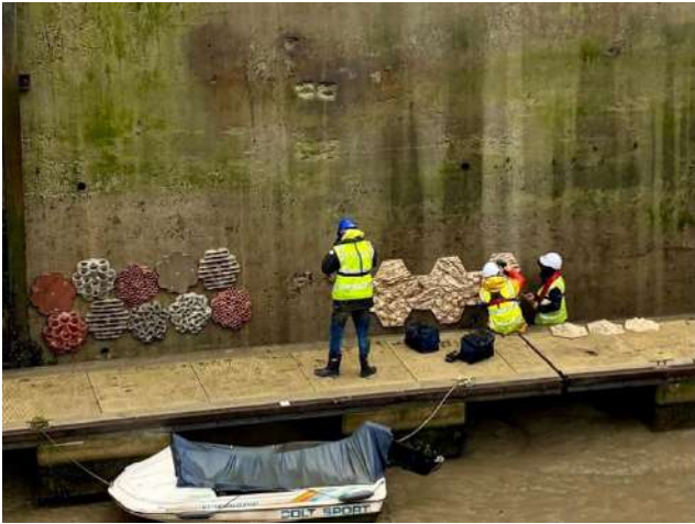
Figure 7.17. Panels being established in Padstow Harbour in November to create a 'Living Sea Wall'. Image: OurOnlyWorld.
